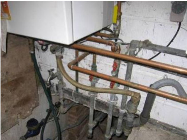
Manglende isolering
